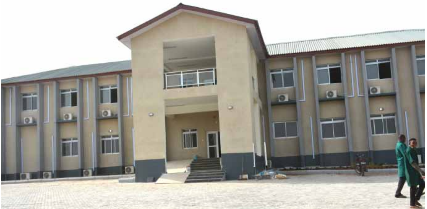
The new Agriserve Building
