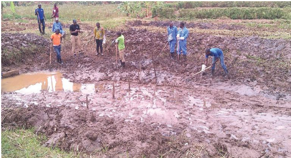
IKYA team excavating their first pond
